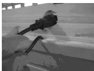
FIG-11 Leading the wires of heaters onto the board through the corresponding hole
