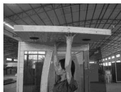
FIG-10 Setting the top board
